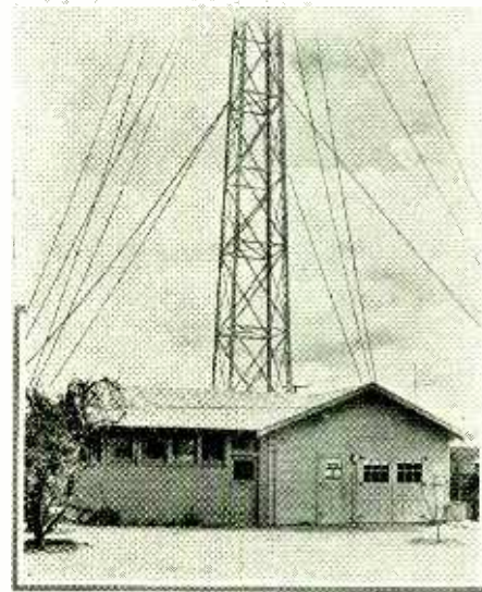
General view of the transmitting station with part of one of the antenna towers in the background.
